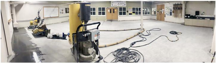
(Above) Phase 1 of the Senior Capstone Design Suite renovation includes cleaning and repolishing of the laboratory floor. Removal and rearrangement of ceiling ductwork is currently underway. (Below) Phase II will include adding more windows.
