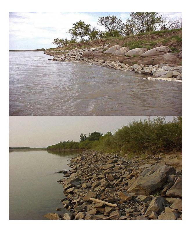
Figure A2-7. Riprap and bank stabilization restrict river function.
