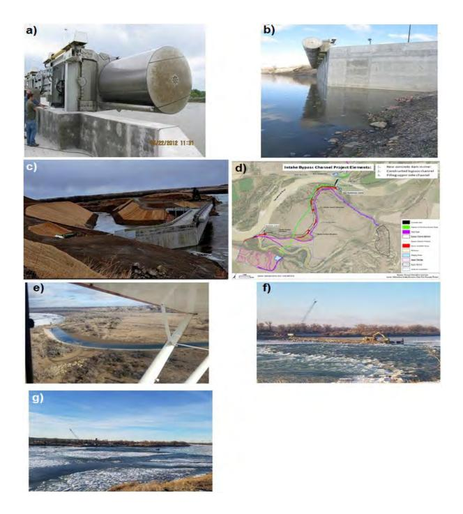
Figure A2-9. Fish passage project improvements at the Intake site - pictures a, b, c: new Intake Canal head gate and screens completed in 2014; d) design elements of project; e) downstream portion of the constructed bypass channel March 2020; f) construction causeway removal after completion of the south half of the new concrete weir December 2020, and g) completed south half of new weir January 2021.
