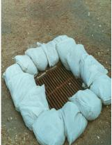
mulated to half the design depth of the trap. All sediments removed should be disposed of properly.
