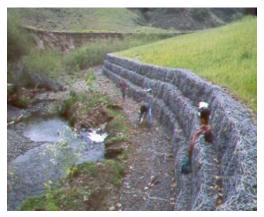
☑ Gabions to be installed in streambanks should be designed and installed according to Rule #9.3 of the Stream Channel Alterations, Rules & Regulations and Minimum Standards, Idaho Department of Water Resources, 1978.
