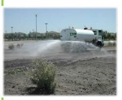
**Sprinkling:** Apply so that the soil is wet but not saturated or muddy and so that air quality requirements are maintained.
