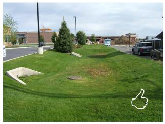
Specifications for swale construction should state the earliest point in construction progress when storm drainage may be directed to the swales, and the means by which this delay in use
