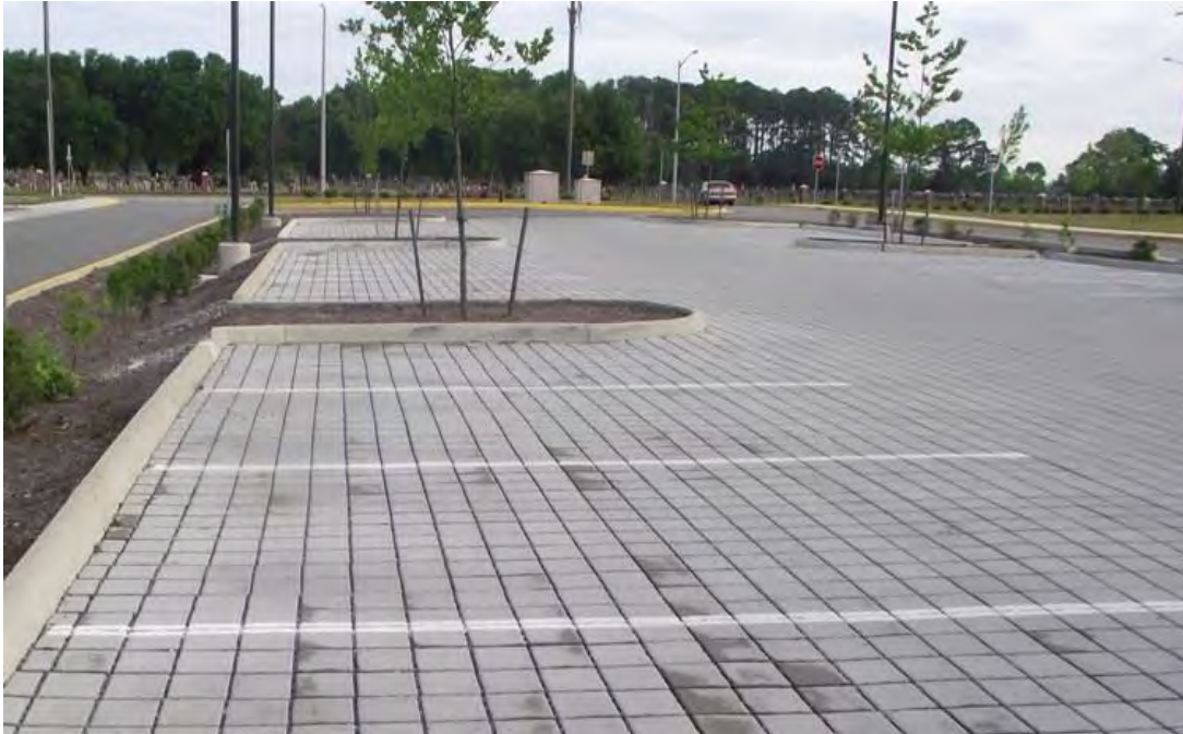
Figure 12. Permeable Paver Parking Lot in Virginia http://www.bractwalls.com/permeable-paver-pictures.htm
