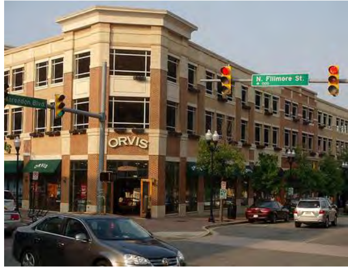
Figure 6. Parking Garage Designed to Blend with its Surroundings: Clarendon Station
